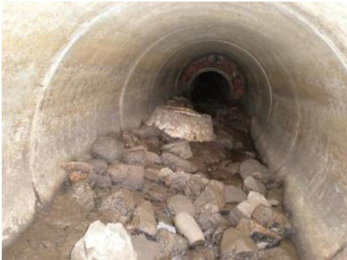
The length of road between the B4069 and the M4 bridge (is this still Church Lane?) had badly blocked ditches, the main culvert under St James was totally blocked (and has been for more than a year) and many other culverts were partially blocked.
