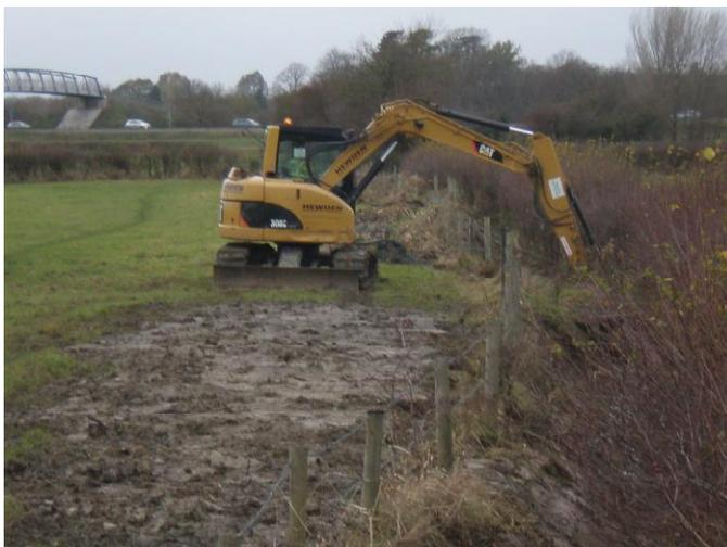
Where The Bourne runs down the western side of to St James to meet Dauntsey Brook, the culvert was far too small... and so presented a flooding risk to St James. A request for a suitable length of pipe that "may be lying about" not only ended up with the pipe, but it installed and this section of main river cleared.
